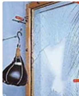
3. Wire-reinforced glass(6.8mm) The wires were cut, and penetrated by the object.
