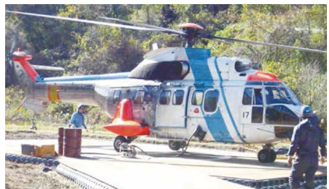
2011: Overhead power cable installation (Fukushima)
