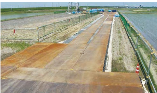
2007: Overhead power cable installation (Niigata)
