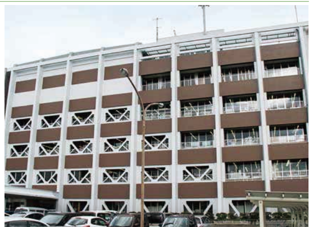
Kashiwazaki City Office (Japan) *Renovation project
