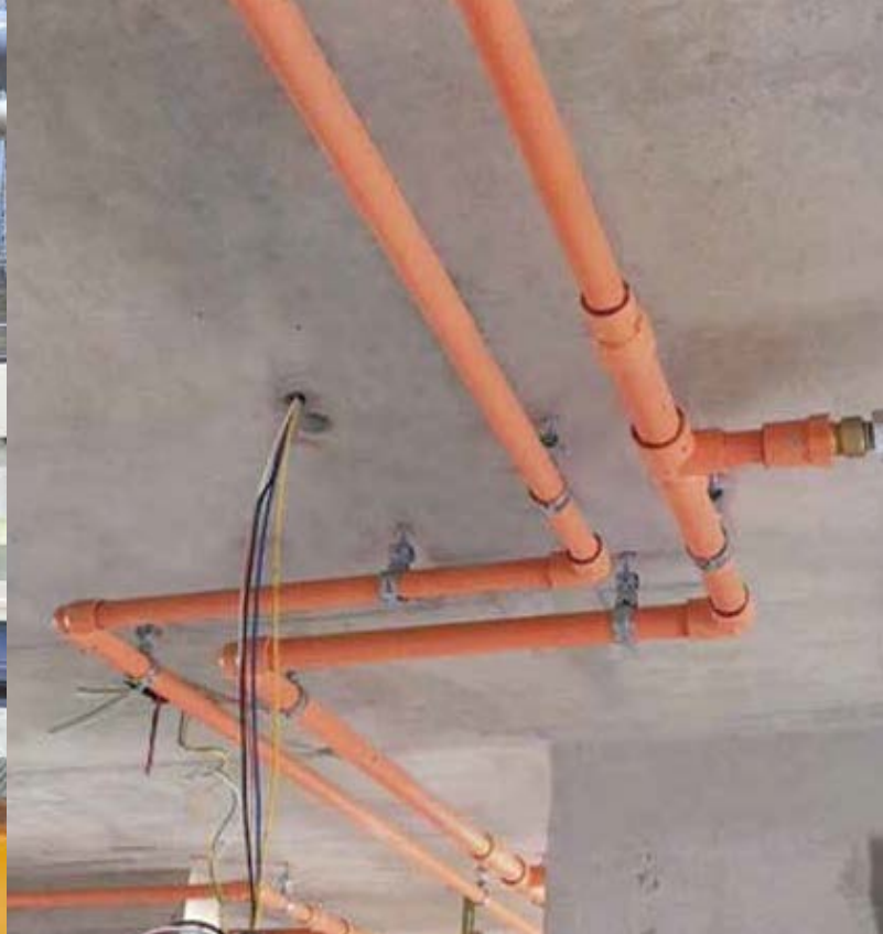
Sprinkler system pipes (superior self-extinguishing properties)
