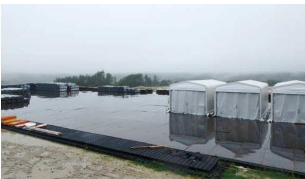
2017: Solar power system installation (Fukushima)
