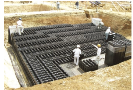
Chiba: Residential land rainwater reservoir (storage capacity: 420m 3 )
