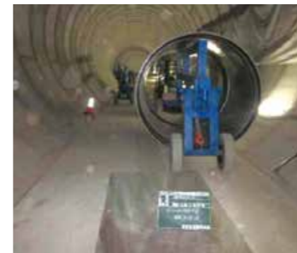
FRPM管運搬
