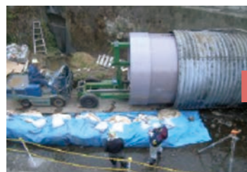
FRPM管運搬
